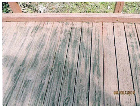
Mold on Deck Boards
