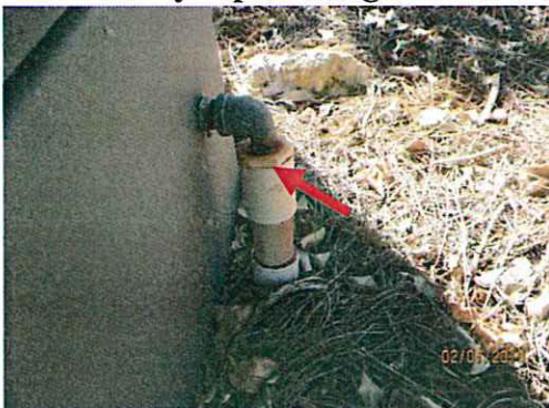
Leaky Pipe Fitting
